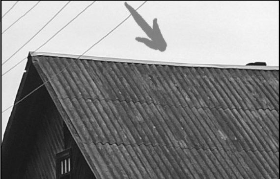
The arrow below is pointing at the metal strip on the ridgeline which repaired the hole.
